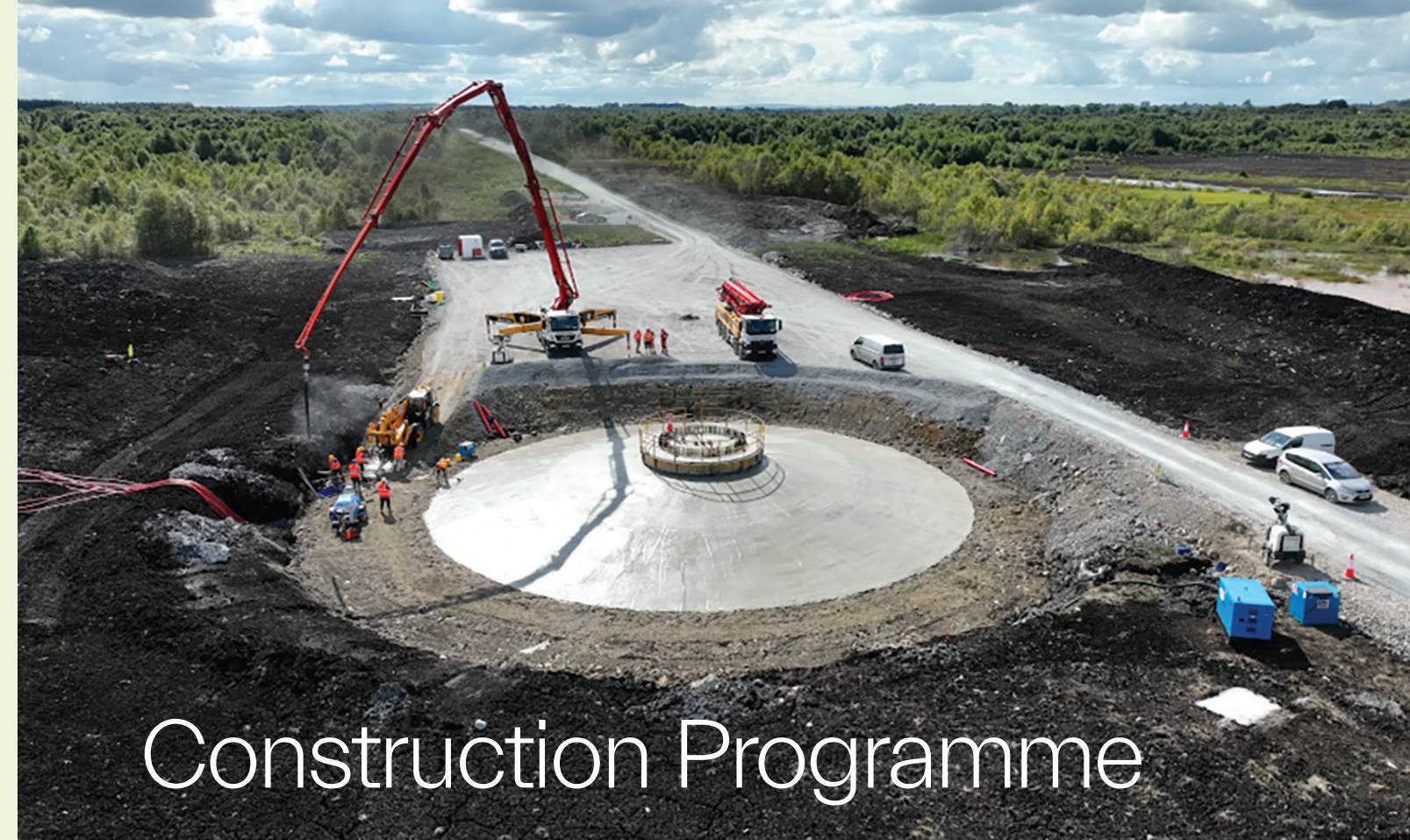
Completed turbine foundation base
