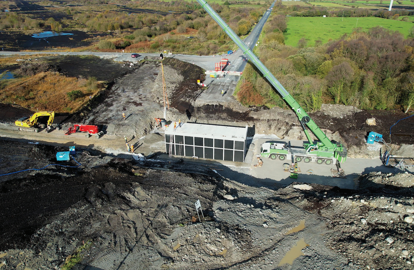
N62 Underpass works under construction, to provide an operational and amenity link between Drinagh and Clongawney bogs.
