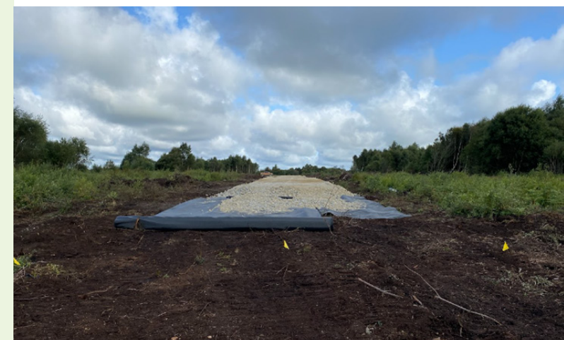
Floated road construction toward Turbine 11.
